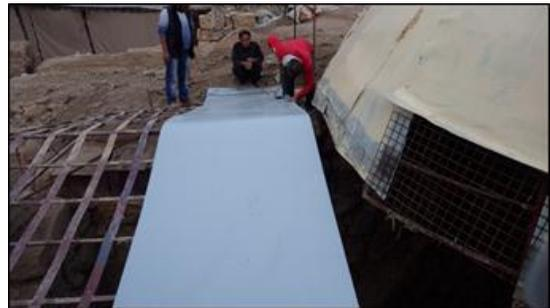
The next stage was in 2014, when we turned our attention to the Abi entrance. The entrance was then also covered with a metal grid that was fixed and welded, then covered with overlapping metal sheets.
