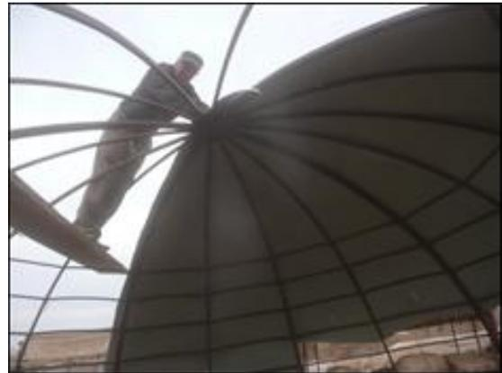
The dome was covered with the metal sheets, and the gaps between the sheets were filled with silicon to maximize the protection.
