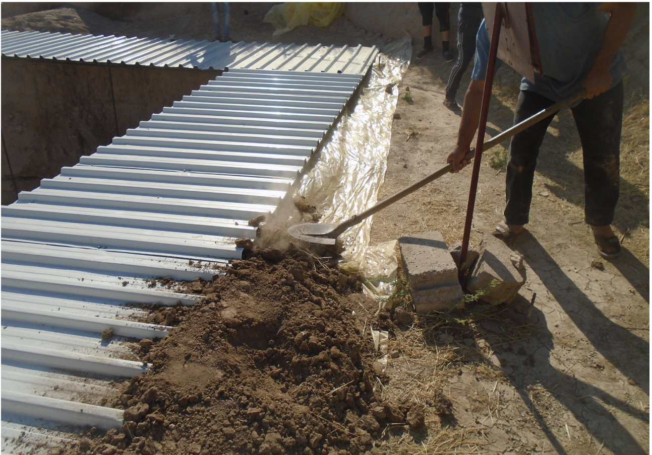
Fig.28 . Covering the edges of tutia with soil - the unit J1
