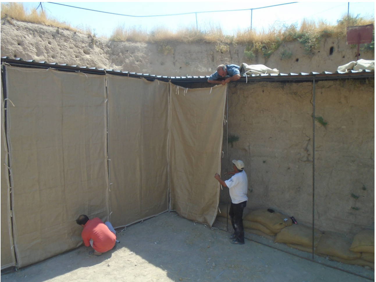
Fig.32 . Fixing the curtain on iron rods by ribbons - the unit J1
