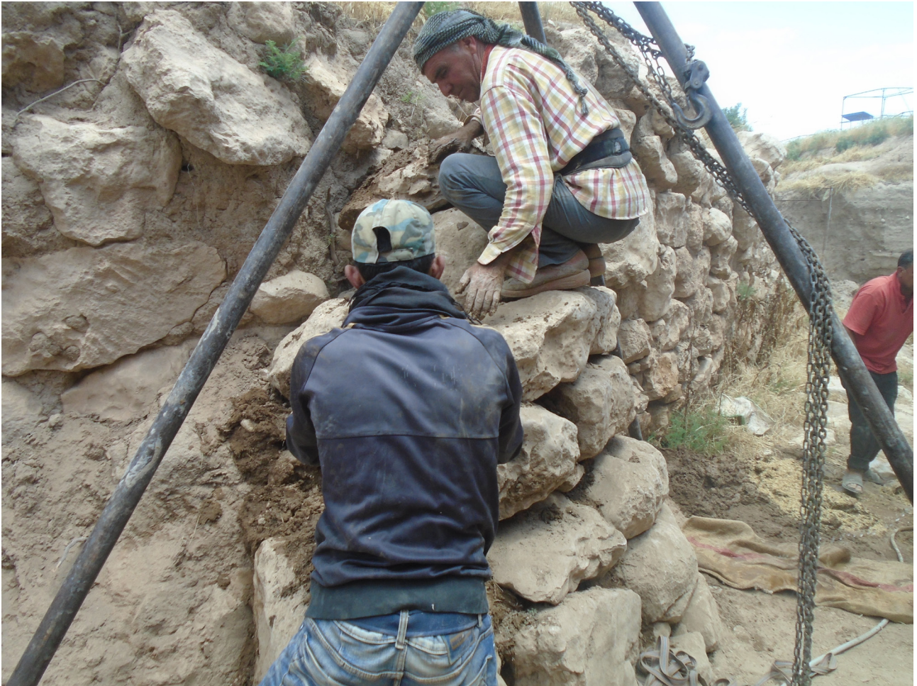
Fig.8 . Filling the gaps between the stones with mud - the unit J5
