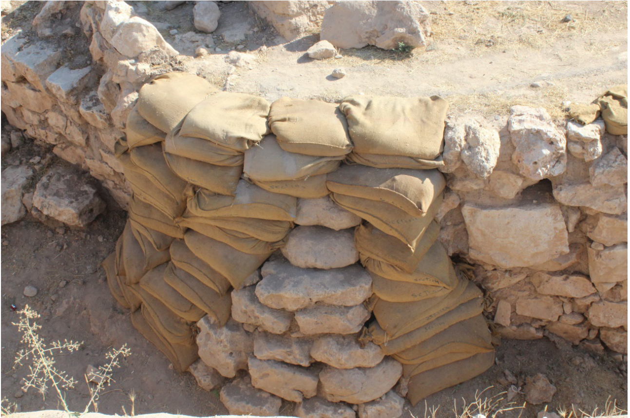
Fig.21 . The new buttress - the unit J5
