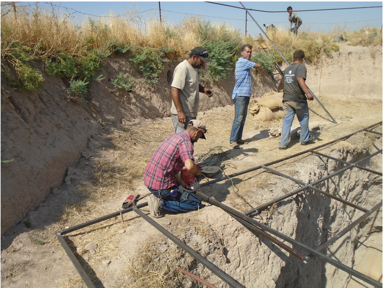
Fig.24 . installing the iron rods - the unit J1
