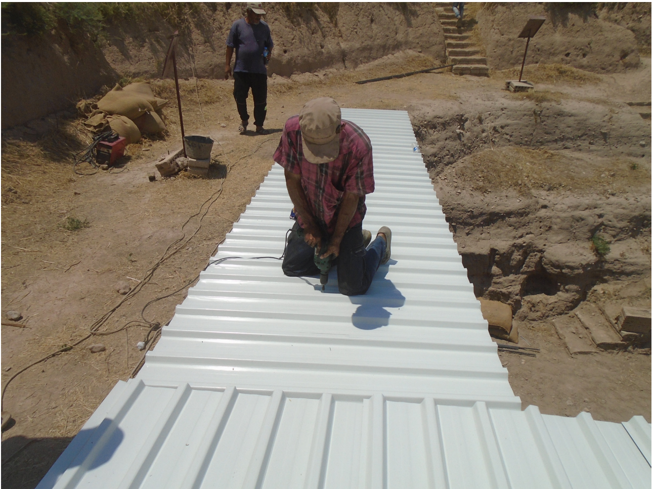
Fig.25 . Fixing the tutia with the iron rods - the unit J1
