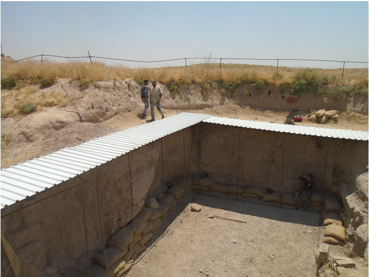
Fig.27 . Iron rods and tutia secured in place, in the unit J1
