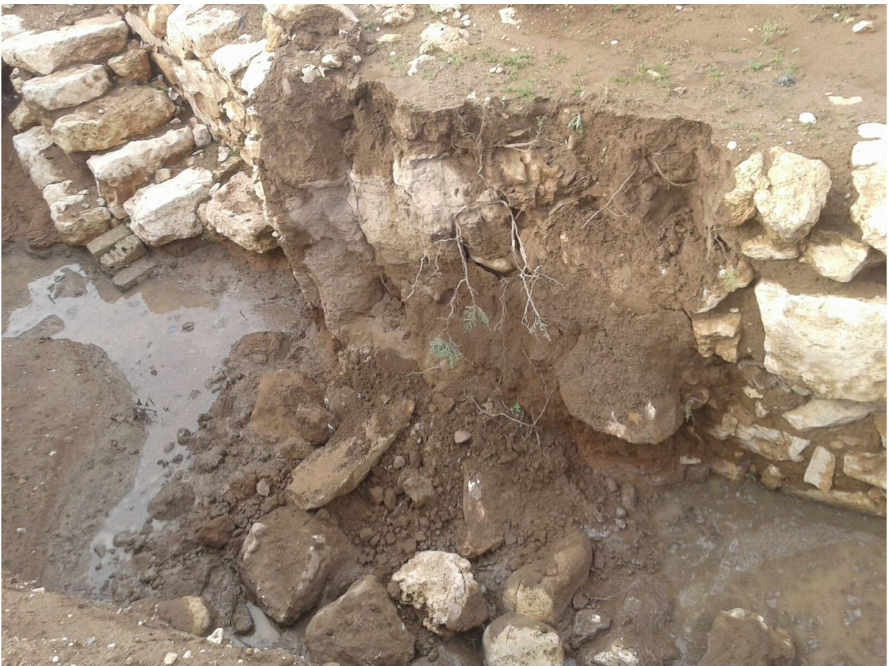
Fig.1 . The crumbled buttress in the unit J5
