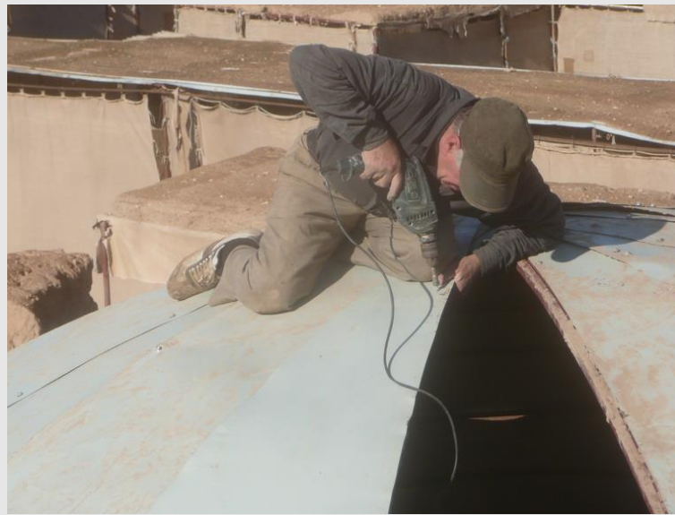
Securing the metal sheets
