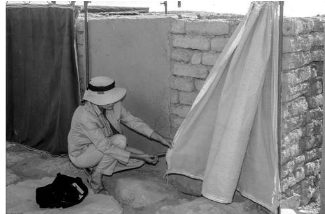
Fig. 6. The aerotextile recommended for trial being held up on one of the test walls.
