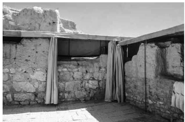
Fig. 4. The protective curtain open for inspection and photography of the walls.
