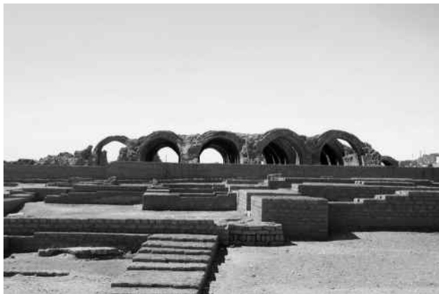
Fig. 1. An example of encasing ruined mudbrick walls with new mudbrick is seen in the Ramesseum on the West Bank of Luxor, Egypt.
