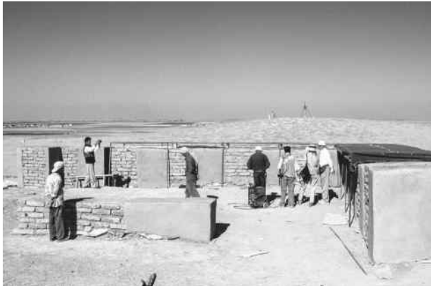
Fig. 5. Test walls, seen here during construction in 2004, were established for comparative evaluation of materials and methods of protection.
