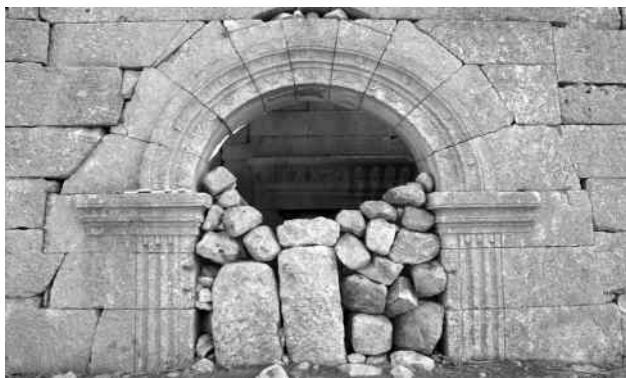
Fig. 19. The entrance of the House no. 25
